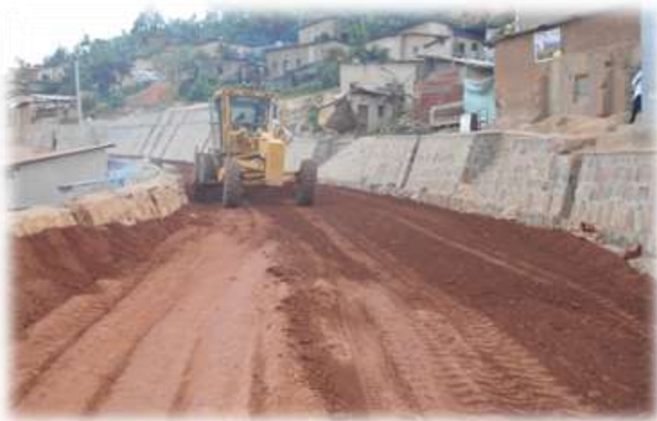
Figure 4.3: Spreading of the backfilling materials
