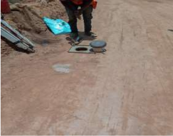
Figure 4.4: Checking the compaction of subgrade by performing in situ density test.
