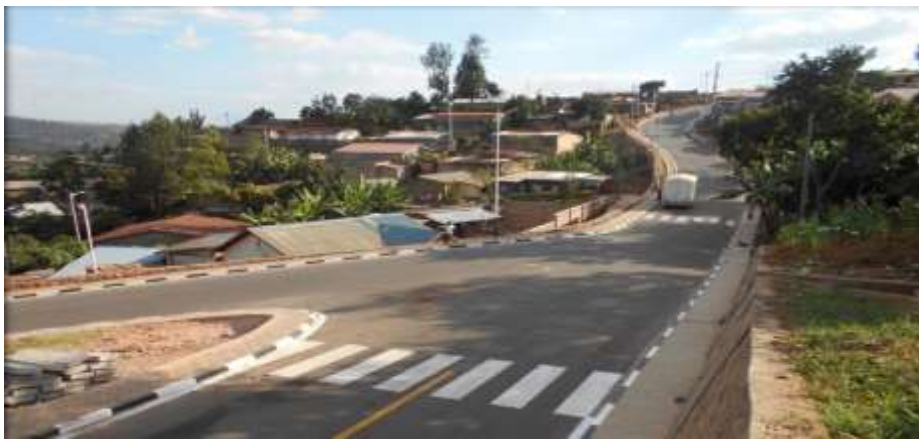
Figure 2.4: A part of AGATARE road construction project at its completion stage
