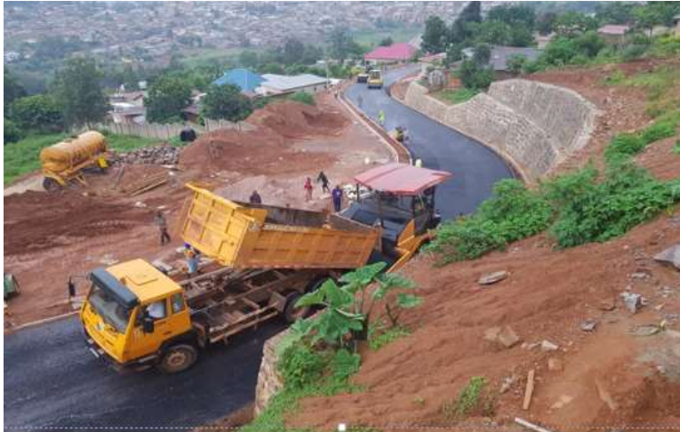
Figure 4.9: Paving asphalt concrete activity, Source: Primary data September 2022
