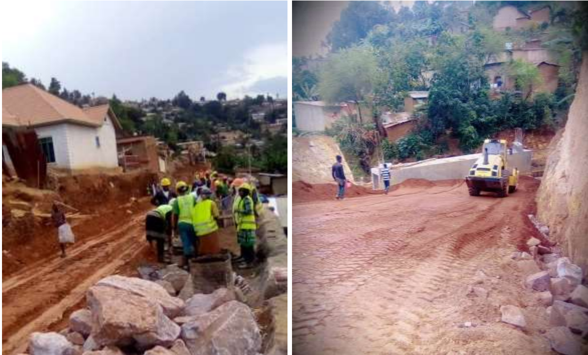
Figure 2.3: Earthworks of cutting and filling Source: Primary data September, 2022
