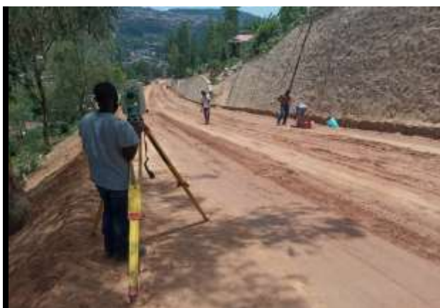
Figure 4.6: Spreading and checking levels of base course materials.
