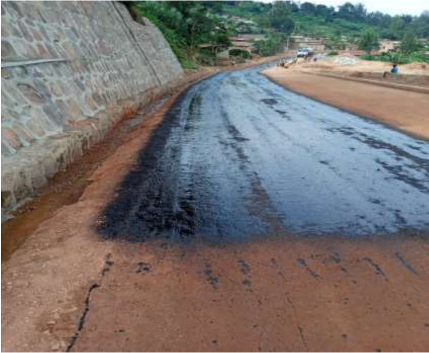
Figure 4.7: Application of prime coat Source: Primary data September 2022
